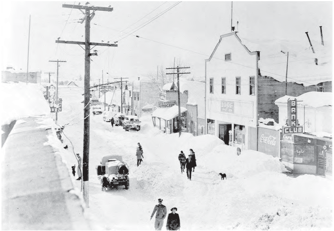
Commercial Street during the winter of 1952, view to west.
