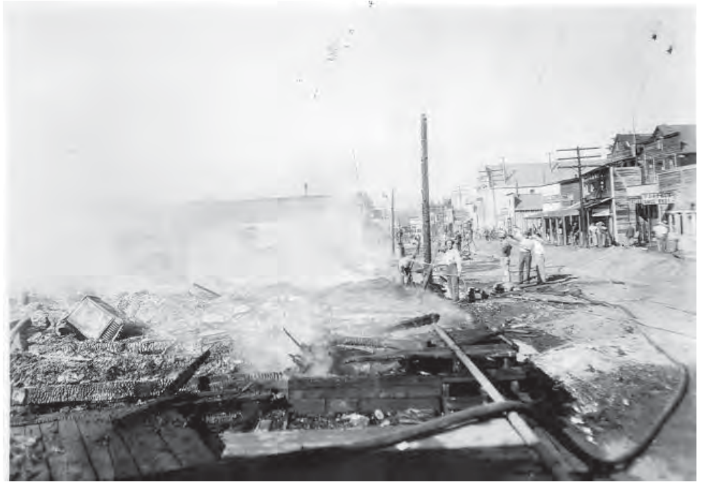
Remains of the south side of Commercial Street on August 24, 1928.
