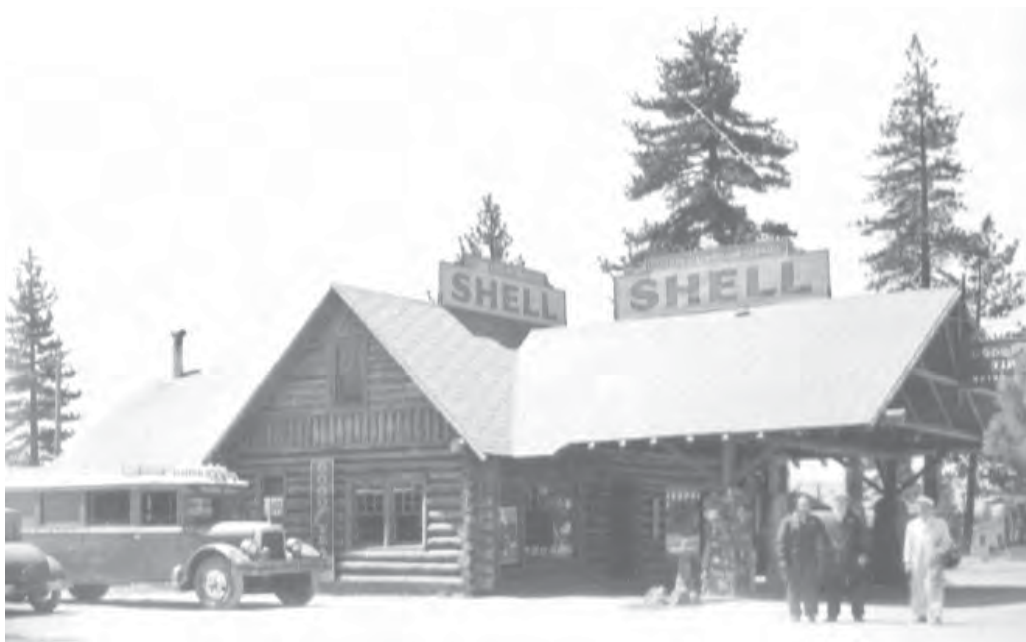
William's home and Shell Station, now the Williams House Museum and Portola Visitor Center, East Sierra Street.
