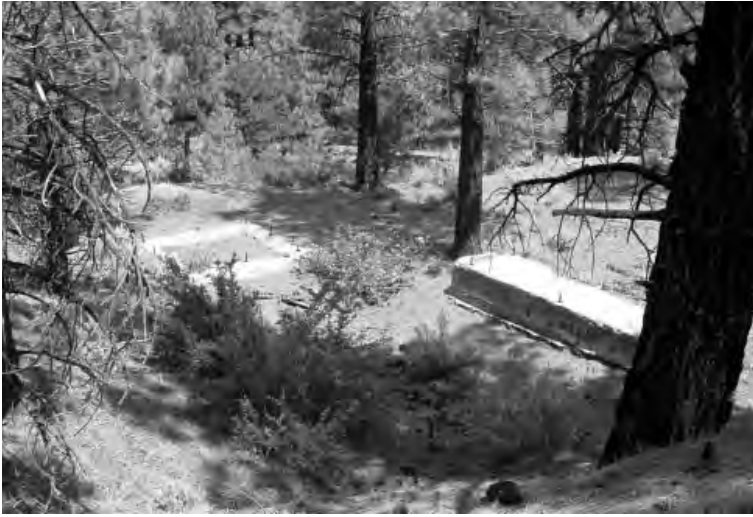
Concrete headframe foundations at the Plinco Mine, 2006.
